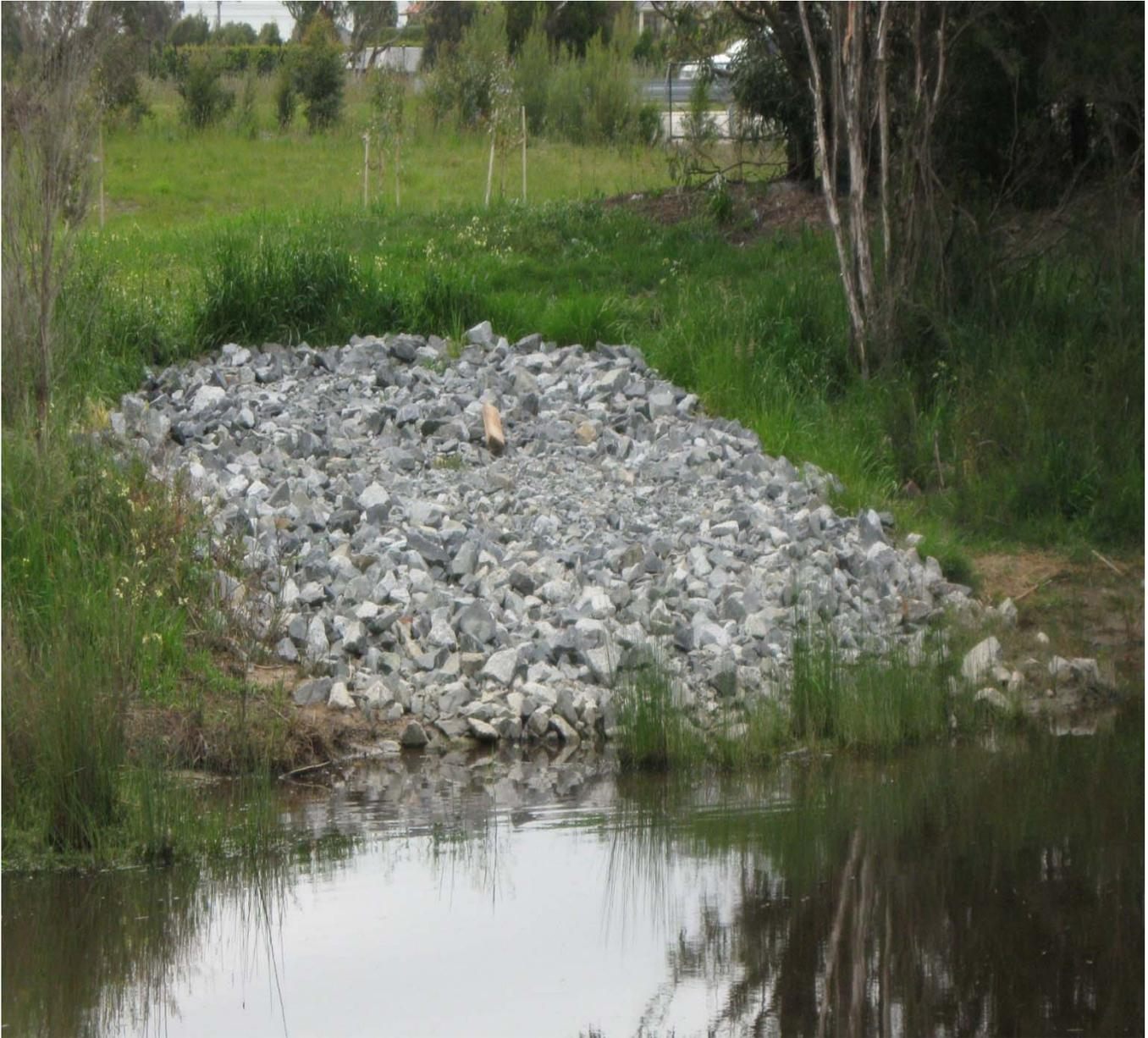
Figure 15: Access track & pond base after rock lining
