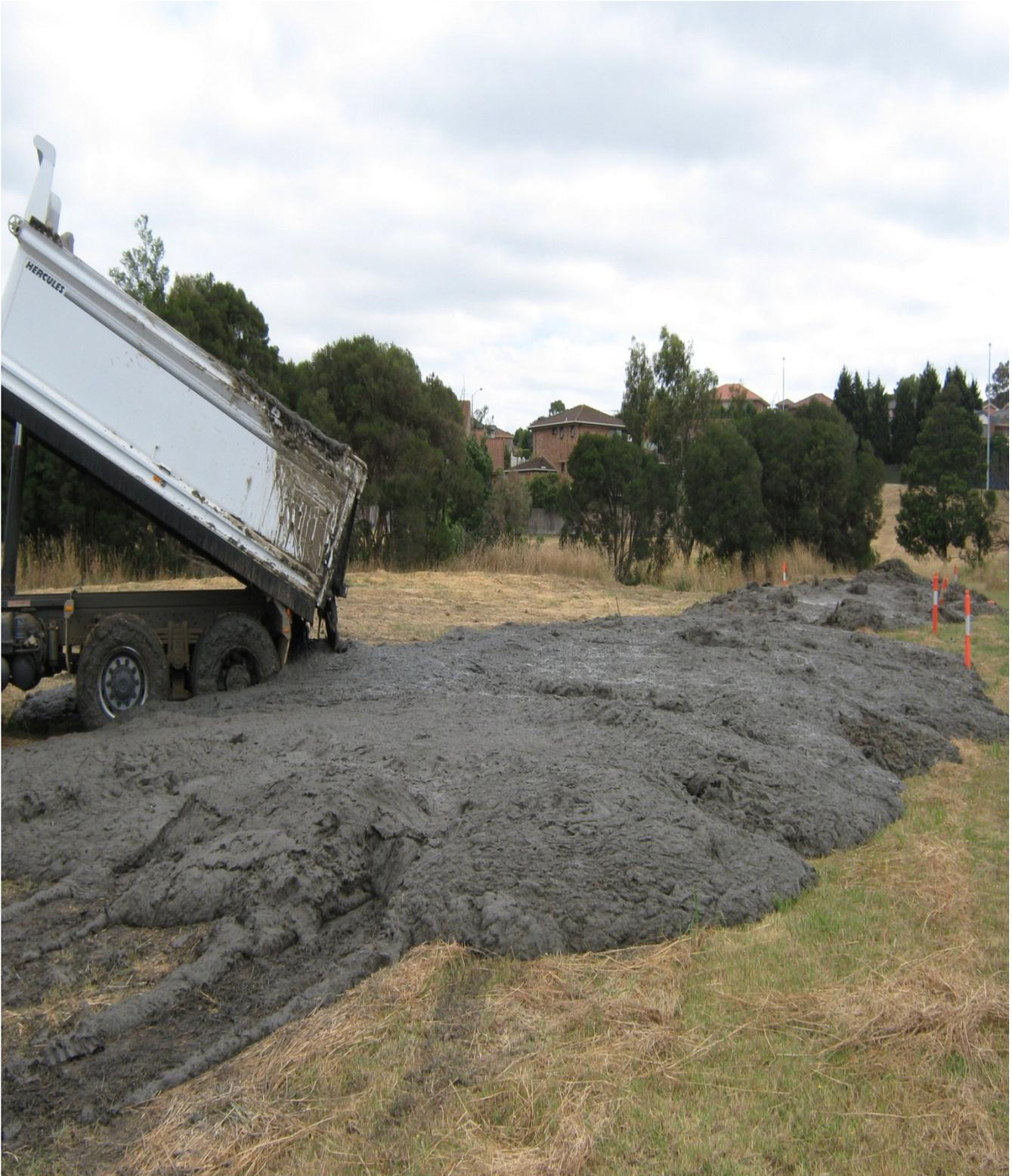
**Figure 11: Material being stacked approximately 150mm high due to consistency**
