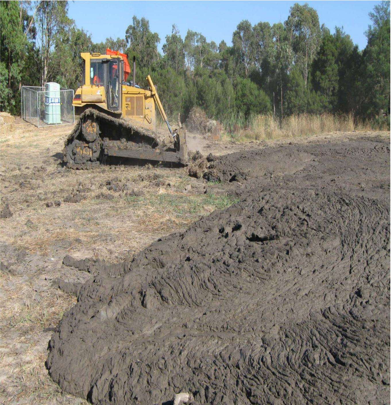
**Figure 13: Swamp dozer turning sediment to assist dry out**
