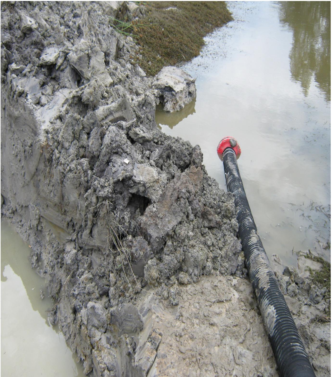
Figure 4: Sediment pond being manually pumped down
