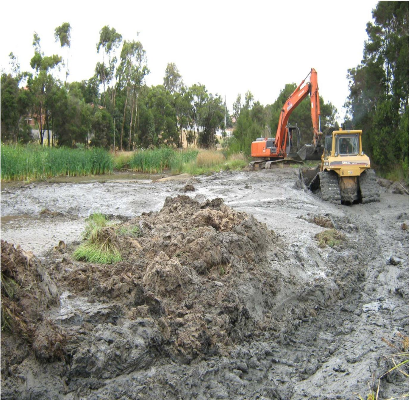
Figure 8: The swamp dozer pushes the semi dried material over to the excavator.
