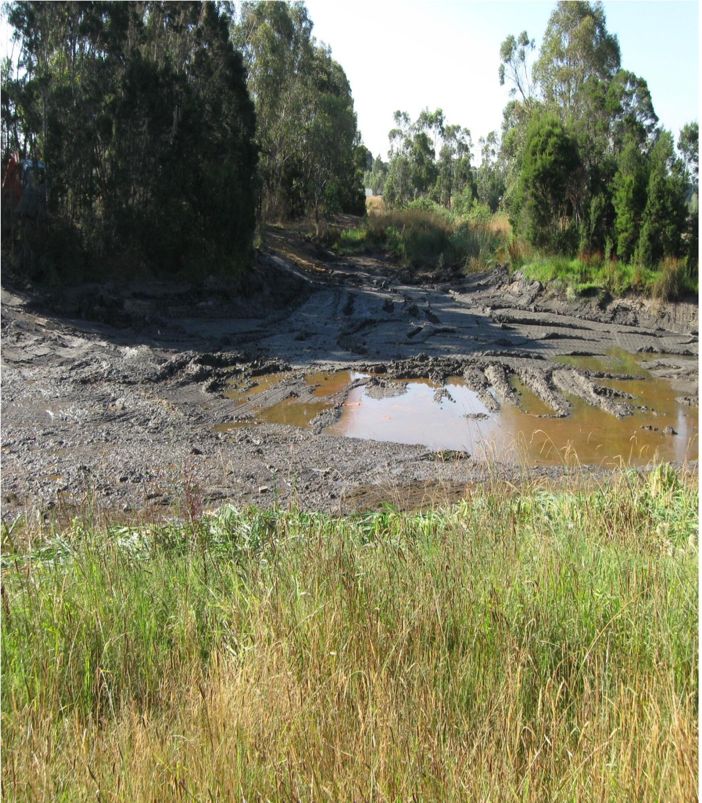
Figure 5: The sediment pond after it has been dewatered.
