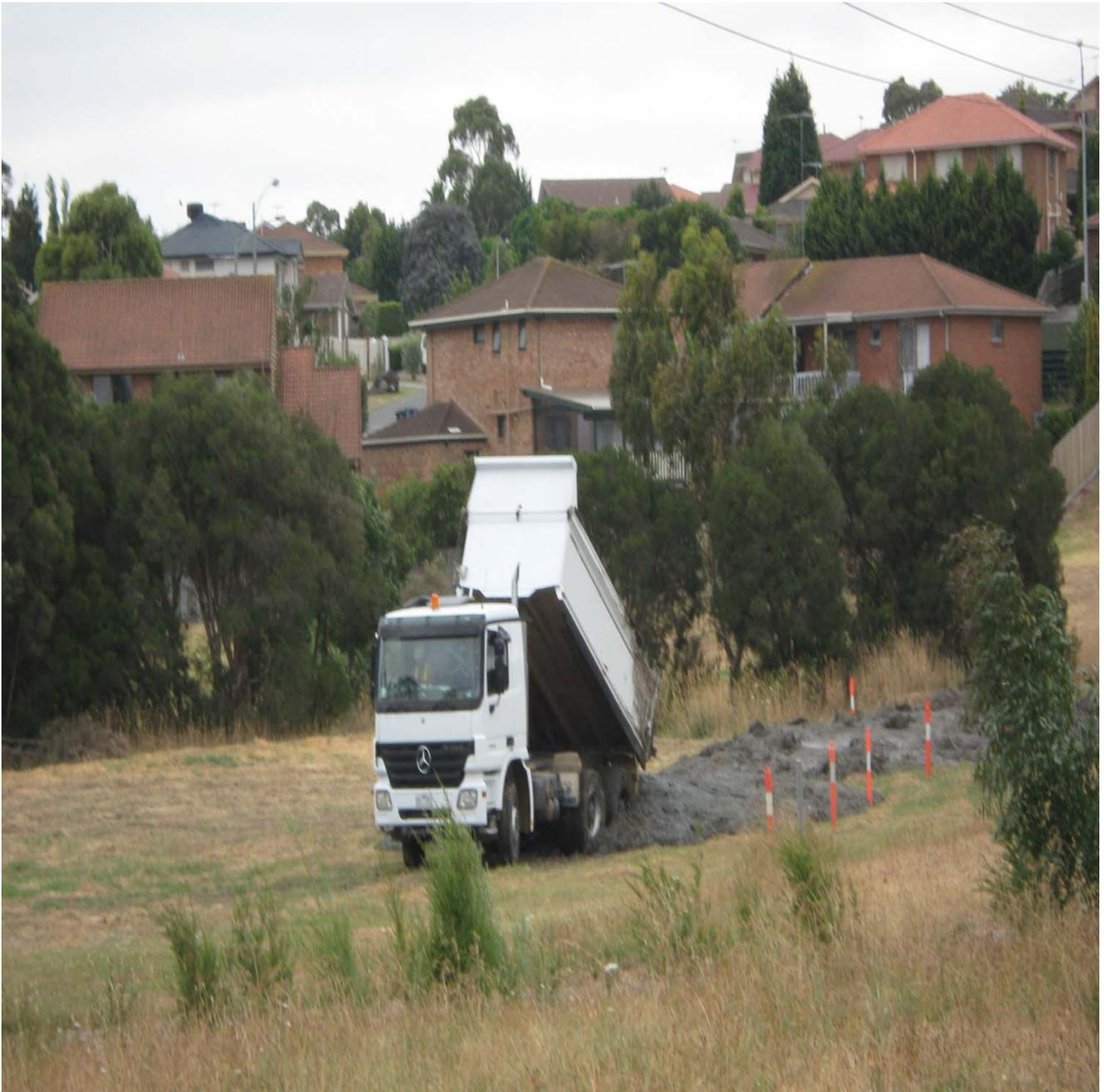
**Figure 10:** Truck depositing material on the temporary dry out area.
