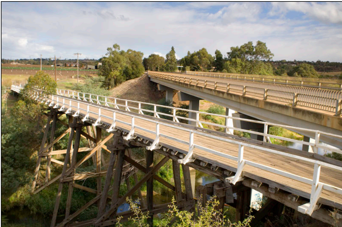
Bridges at Arundel Weir Keilor
