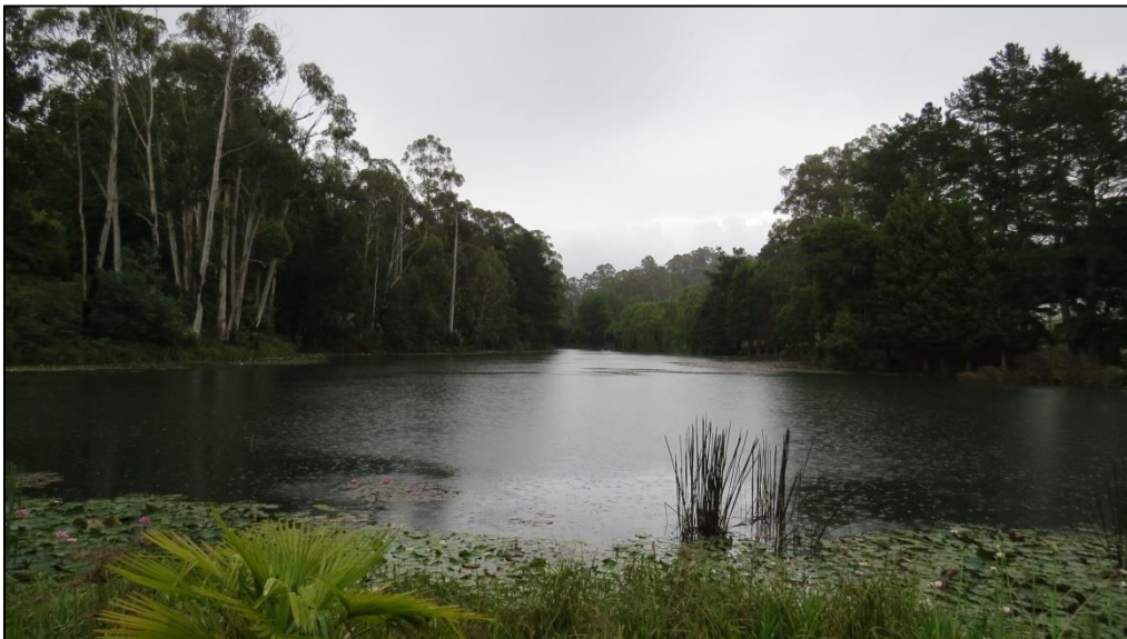
On-stream Dam Ferndale Creek
