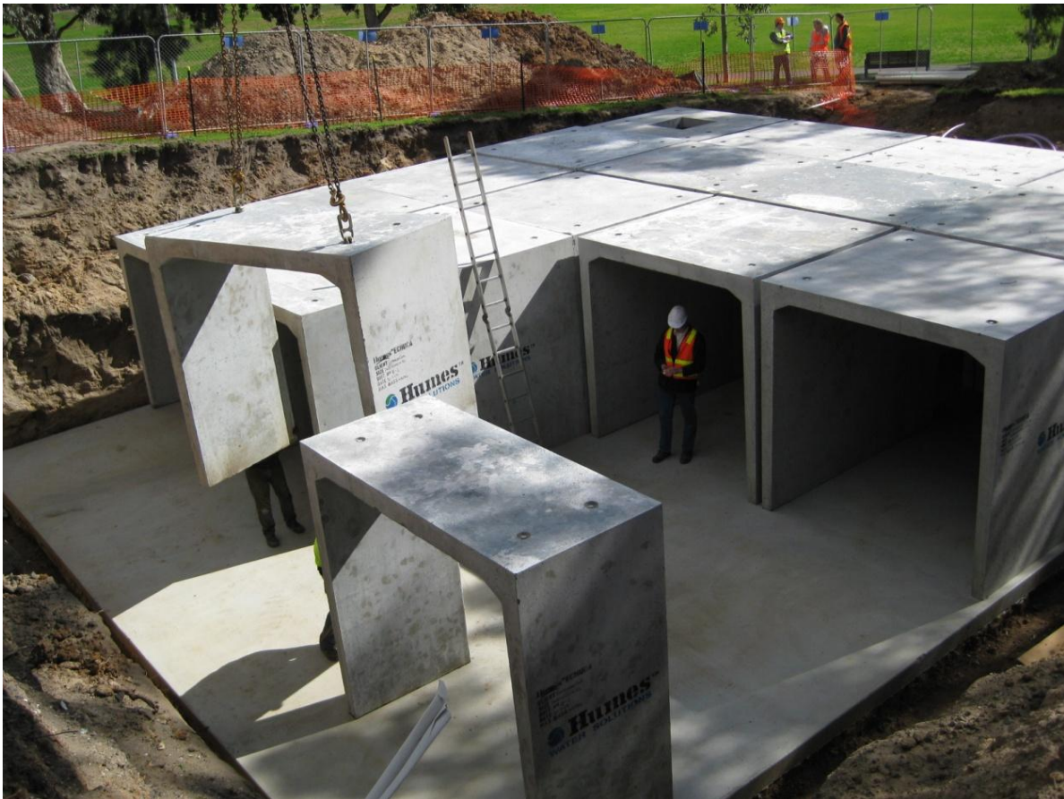
Figure 14 Construction of underground storage
