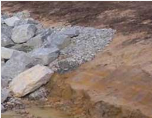
✓ Coarse grade filter/embedment material under lining rocks.
