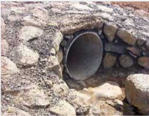
✓ Well embedded rockwork.
