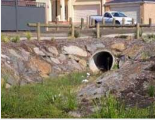
✓ Well embedded rockwork.
