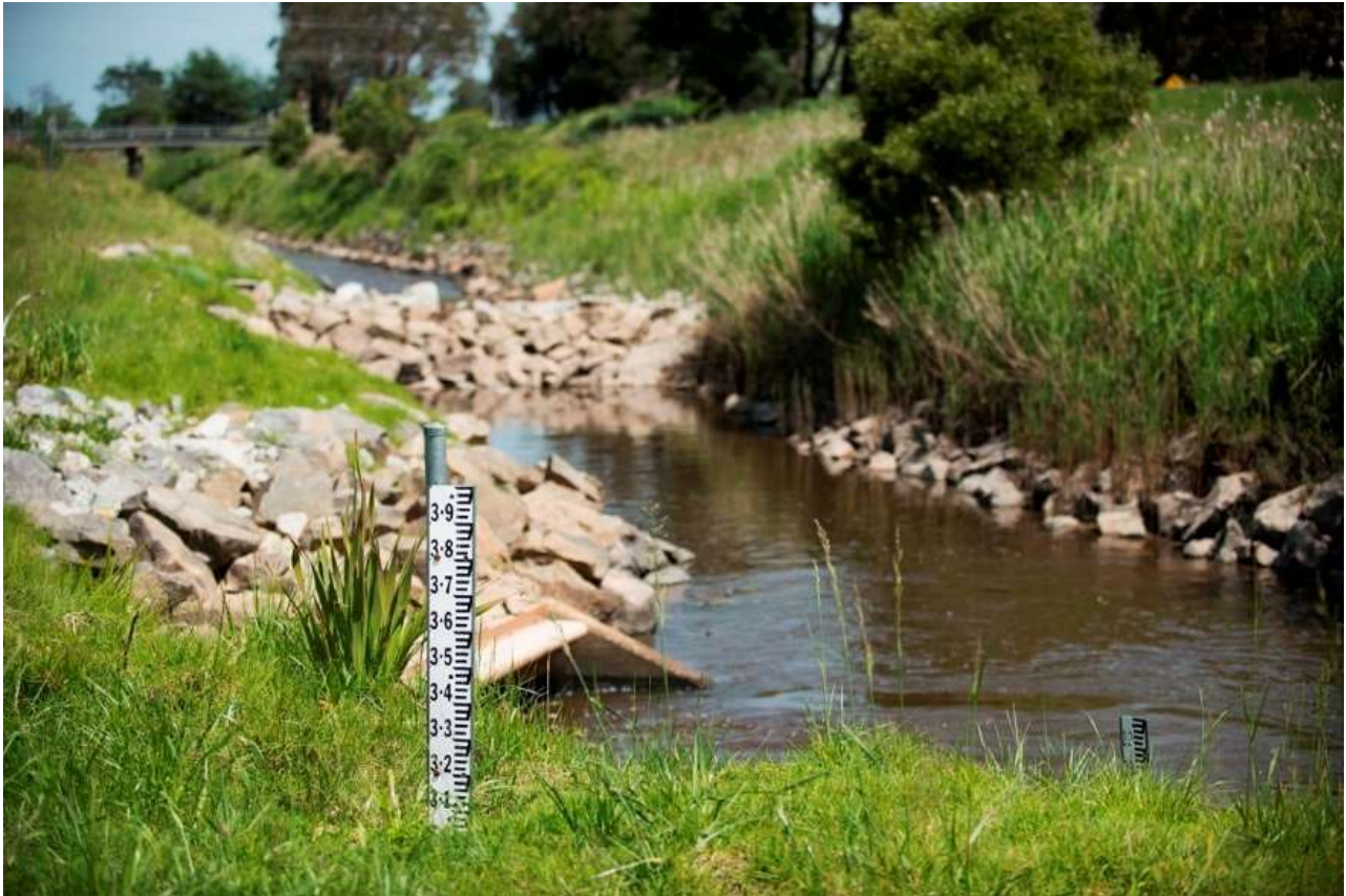
Flow gauge on waterway
