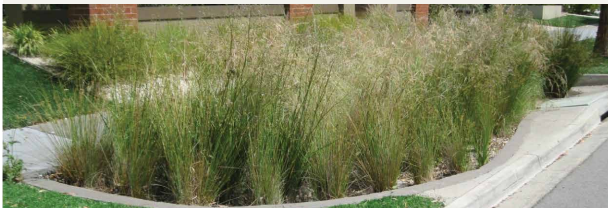
Figure 5 Healthy, densely planted vegetation is important to the long term performance of the raingarden
