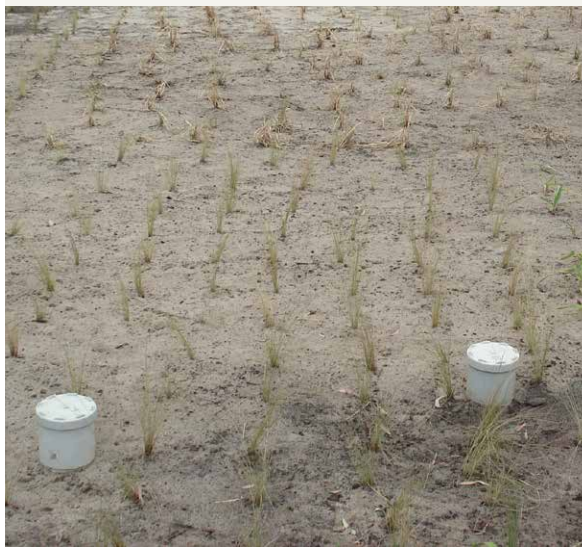
Figure 7 Example of inspection openings in a raingarden
