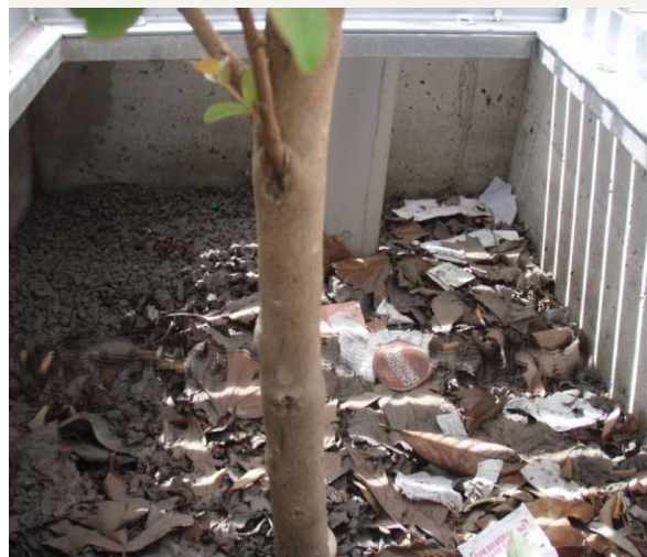
Figure 10 Leaf litter and sediment accumulation in a tree pit located in a busy commercial precinct
