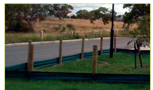
Sediment fence protecting raingarden on a nature strip.
