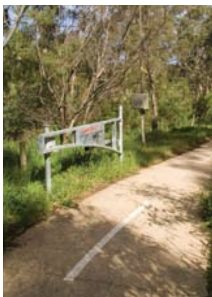
FLOOD ACTIVATED BOOM GATE
