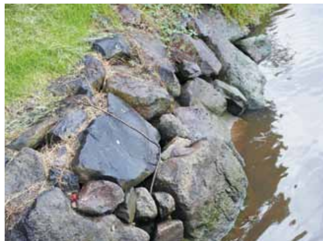
Example of bank stabilisation – Yarra River
