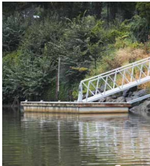
An example of a floating jetty.
