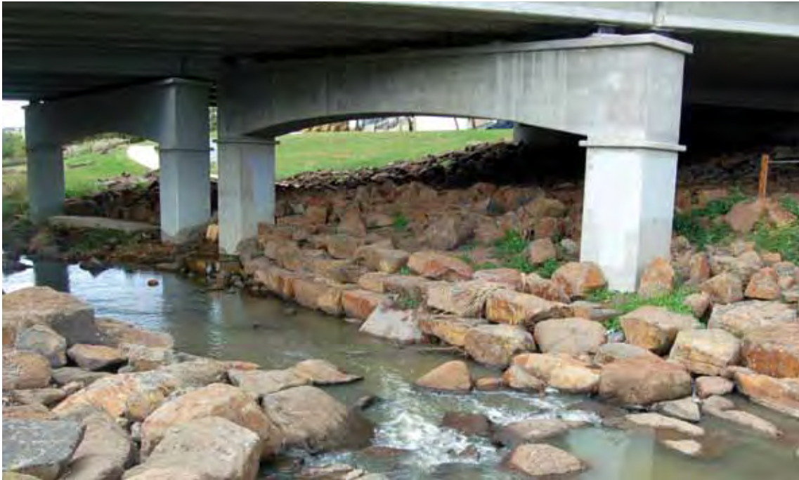
An example of a large single span bridge where the bridge supports are outside of the waterway.
