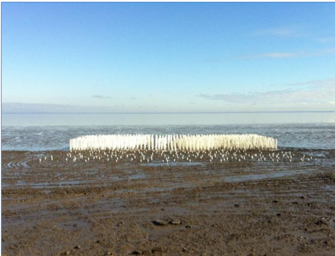
Figure 33: PVC pipe pile field (with experimental plantings in foreground)
