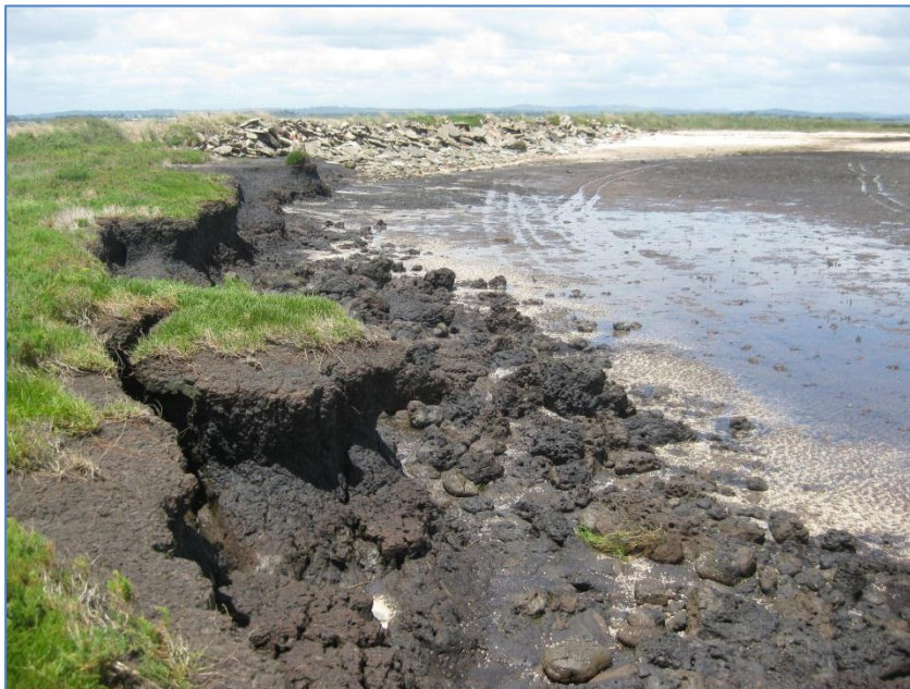
Figure 2: Example of erosion occurring along Lang Lang Coast in foreground with landholder attempts at stabilisation with concrete rubble in background.
