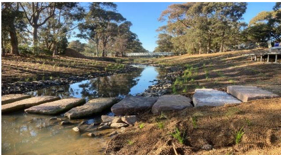
Looking upstream towards new shared user bridge
