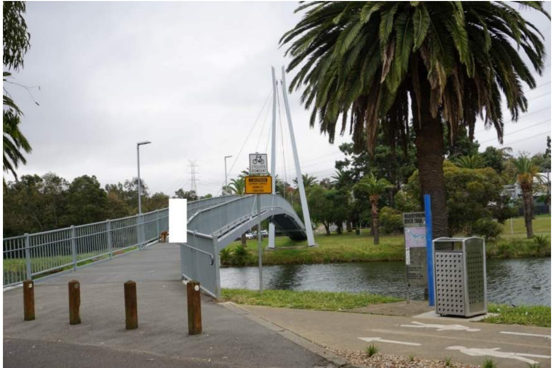
Afton St footbridge
