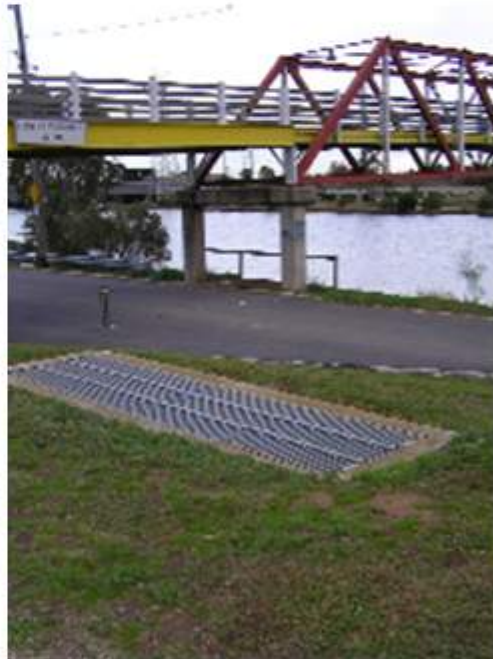
Flood Gates Pit
