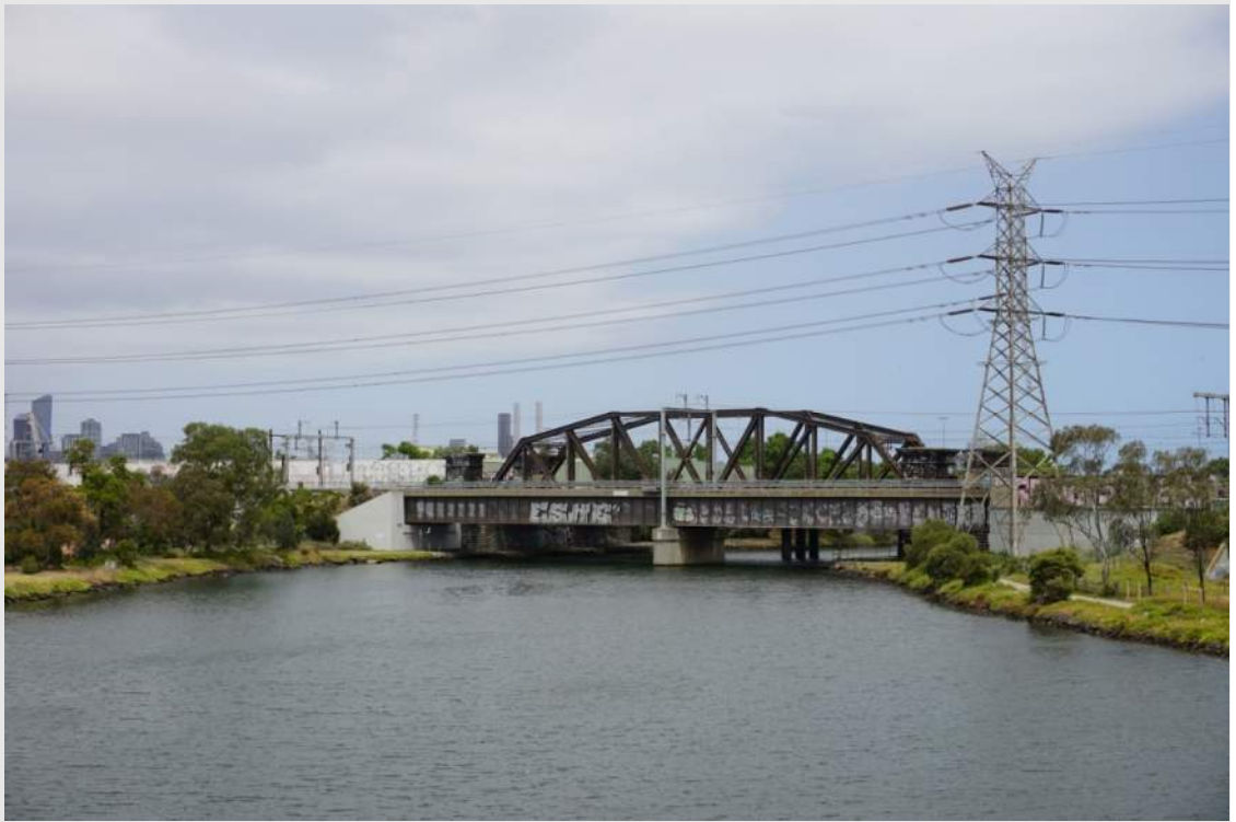
Kensington rail bridge (U/S of the three)
