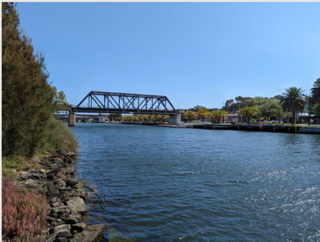
Bunbury St rail bridge
