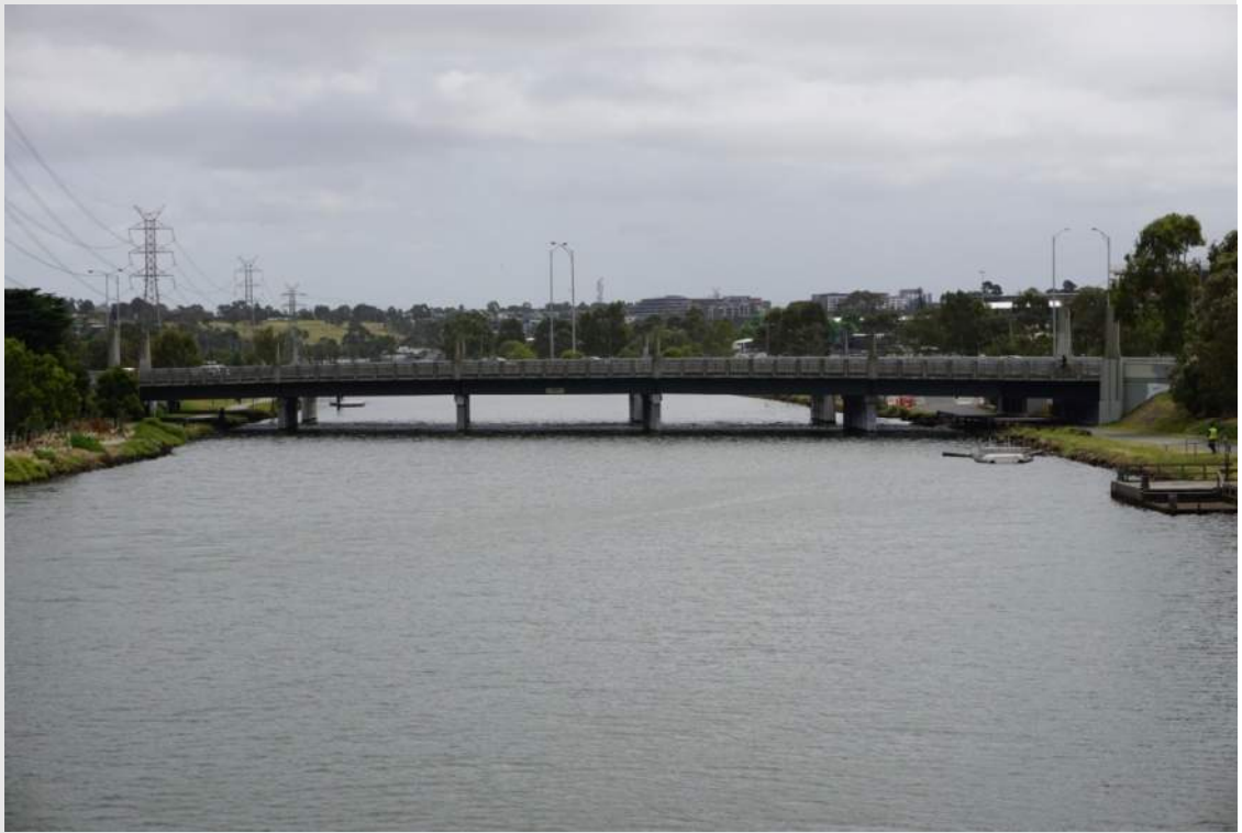
Lynchs bridge (D/S of the two)
