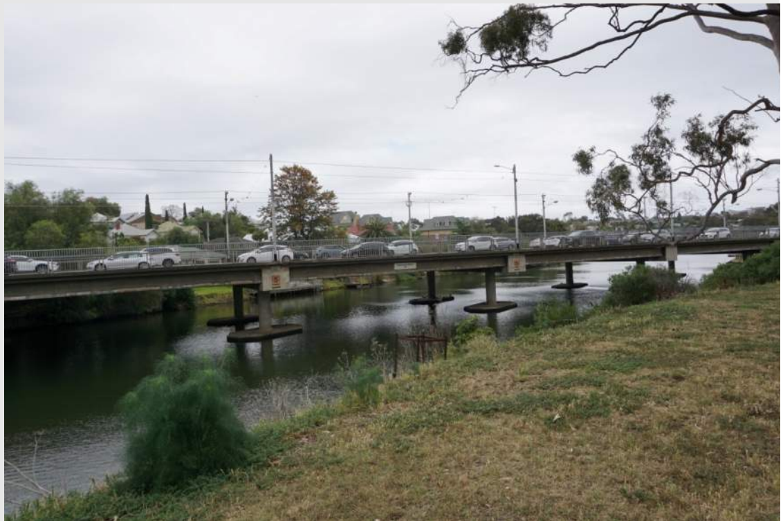
Raleigh Rd bridge
