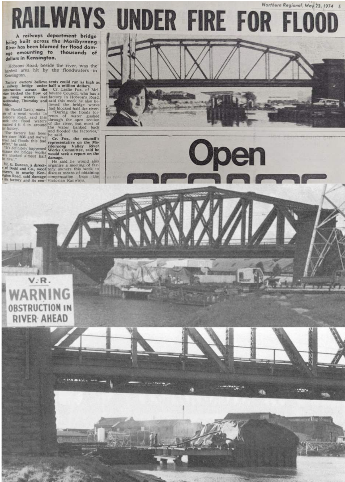
Figure 6-42: Newspaper reports and photos taken in the aftermath of the 1974 flood event around the cofferdam in the river at the Kensington rail bridge obstructing the flowpath thereby likely exacerbating the flood.
