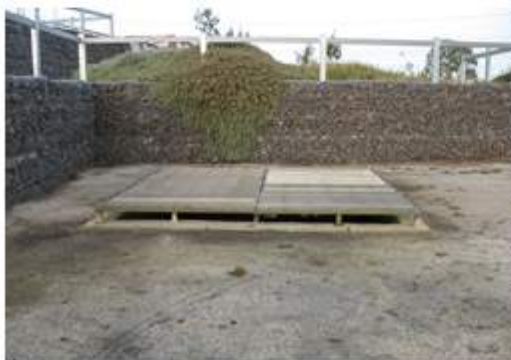
Location of Hobsons Road Trash Rack Pit
