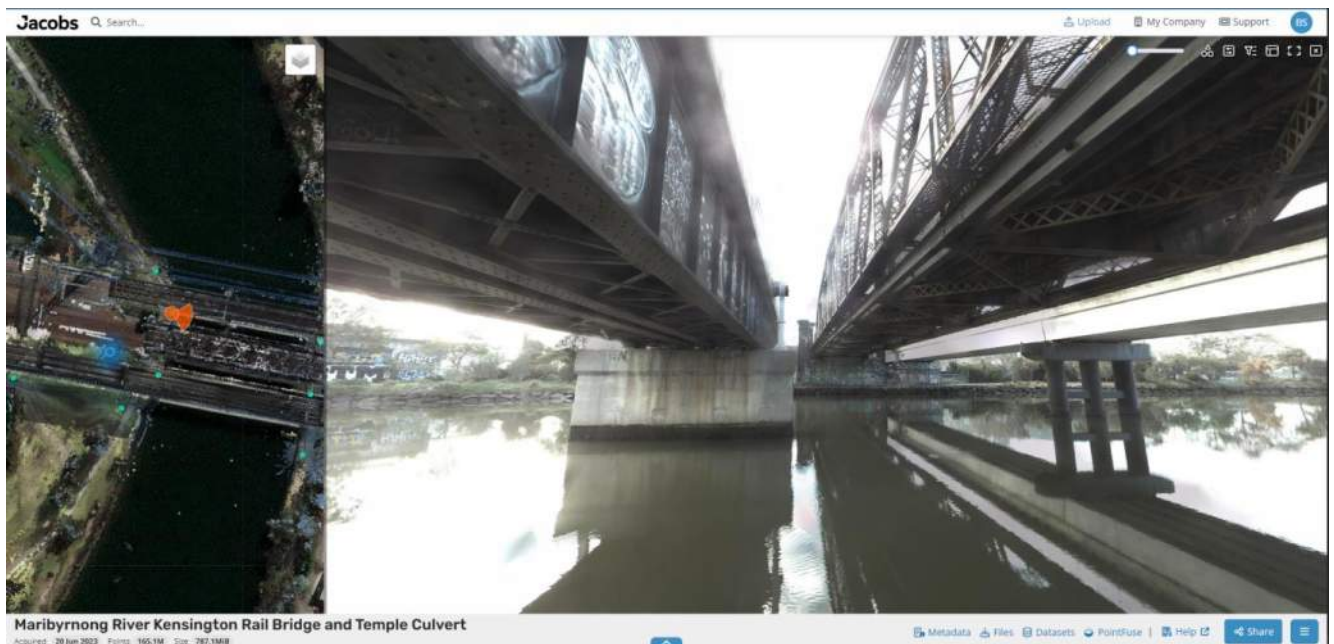
Figure 5 – Pointerra viewer of point cloud and panoramic imagery of Kensington Rail Bridge
