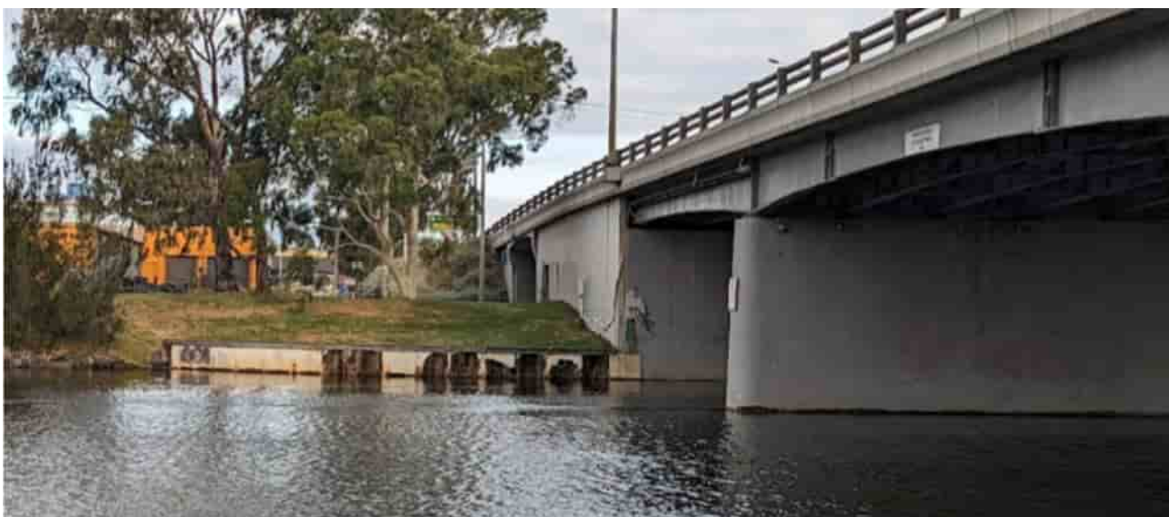
Figure 3-7: Footscray Road bridge from the western bank, facing east where the upstream flow 'training wall' is visible (photo taken in 2023).
