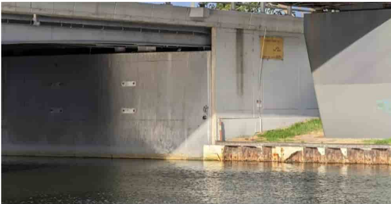
Figure 3-6: Footscray Road bridge from the western bank, facing east where the downstream 'training wall' is visible (photo taken in 2023).
