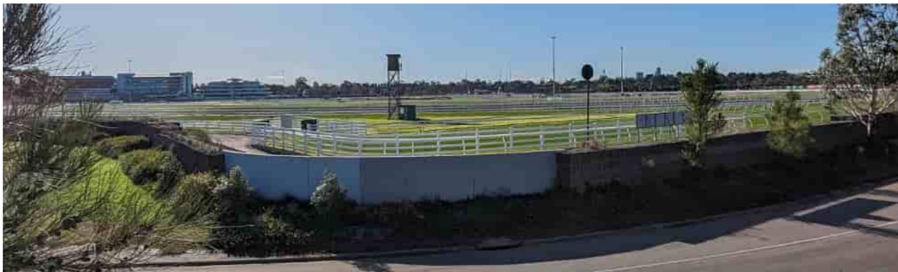
Figure 3-1: Picture of the VRC flood wall taken at the southern edge of the wall, along Chiquita Drive, looking north.
