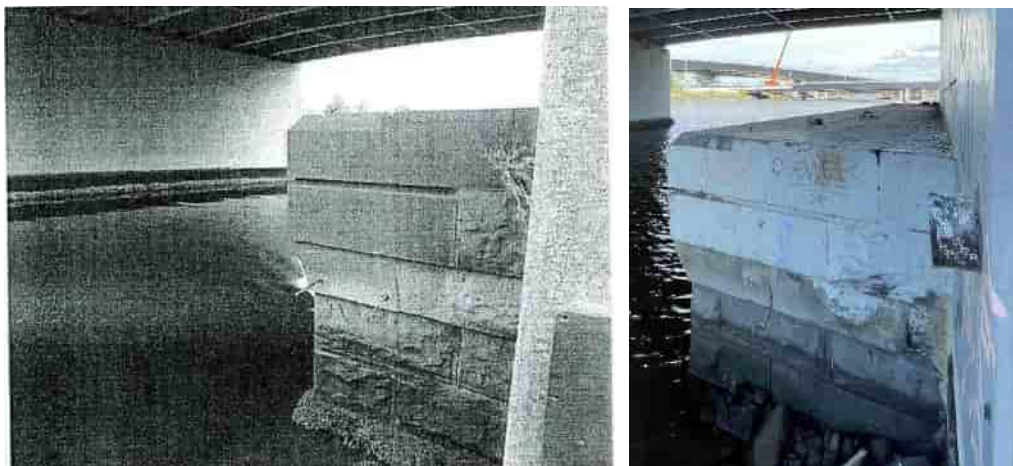
Figure 3-4: Bluestone abutment under Footscray Road bridge on the eastern bank removed as mitigation works (left) (GHD, 2003b) and the abutment that remains on the western bank (right) (photo taken in 2023).
