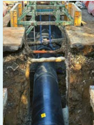
Figure 6. Pipe laid under domestic services.
