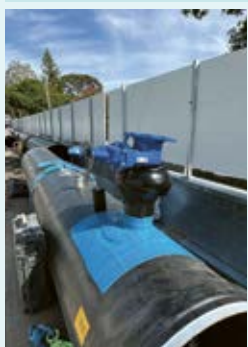
Figure 1. Pipes fitted with valve connection.
