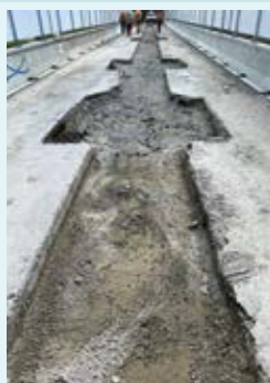
Figure 2. Preparation for asphalt reinstatement.
