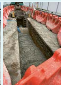
Figure 3. Backfill after pipe installation.
