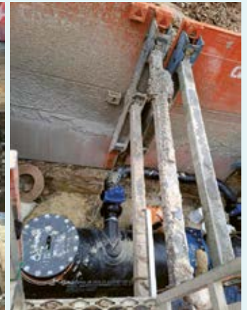
Figure 7. Bypass installation.
