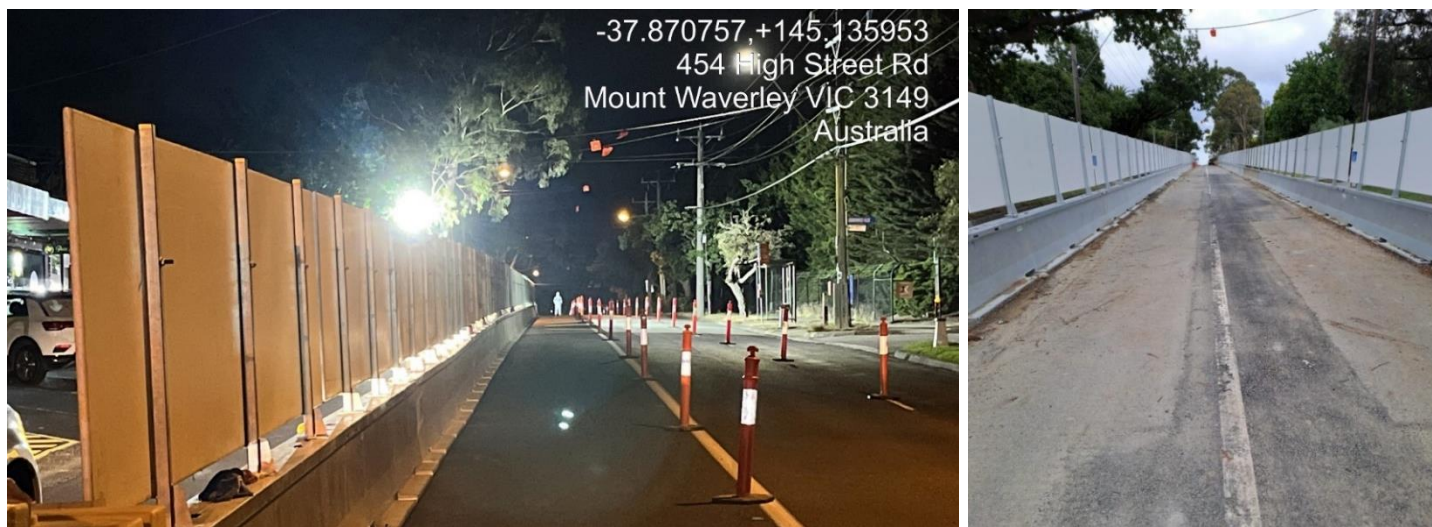
Figure 2-3: Barrier install works at night and barriers on High Street Road
