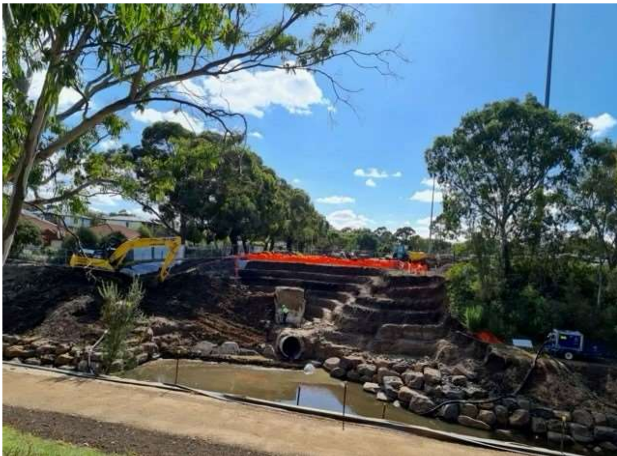
Pond and terracing works in progress
