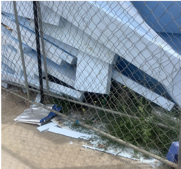
Polystyrene left up against fence, shavings over the pavement. A clear example of inadequate containment (Yarra Riverkeeper Association)
