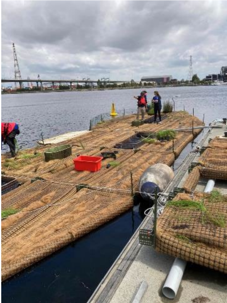
Floating wetlands, preparation prior to installation
