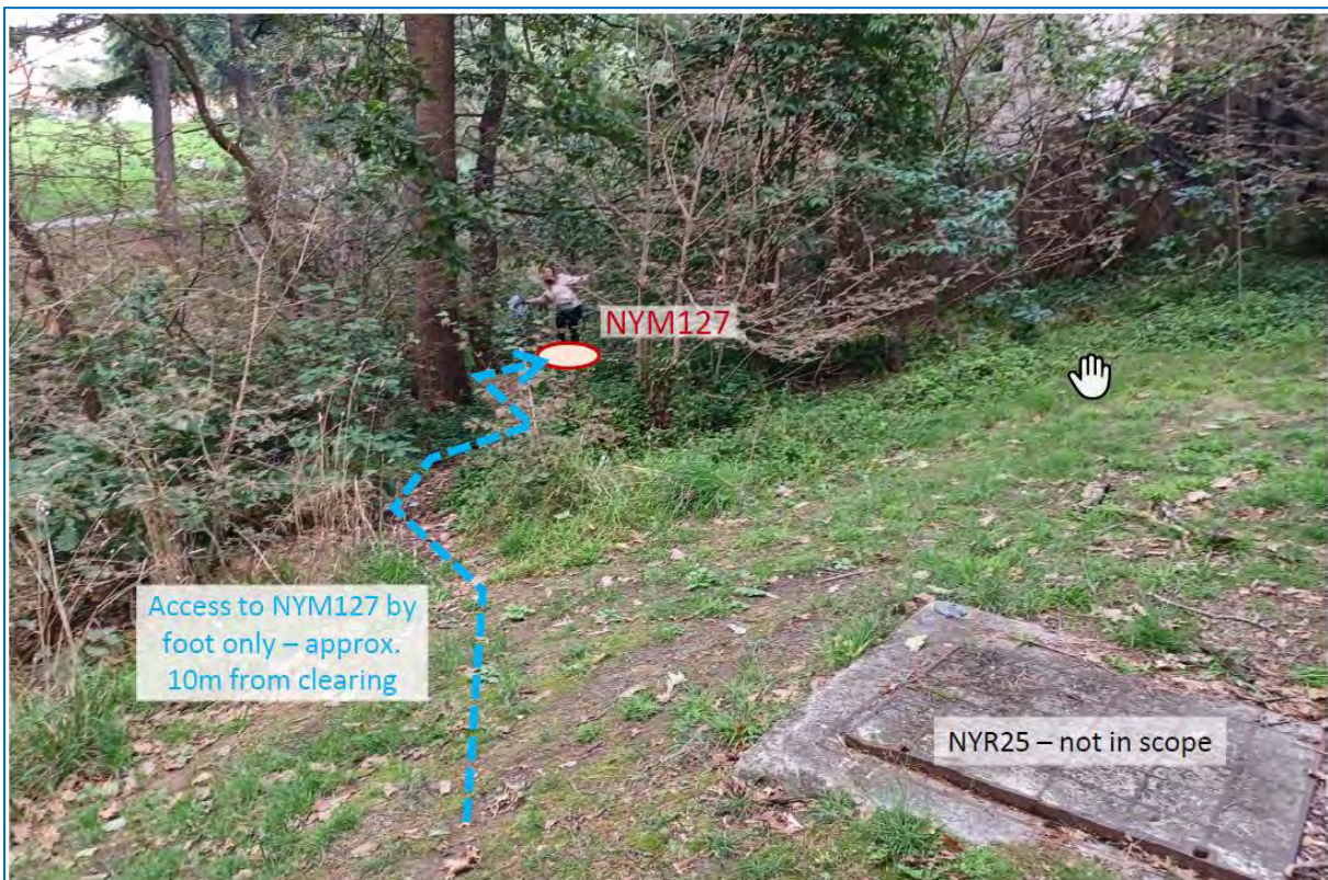
Figure 3 Access widening and small tree removal to NYM127
