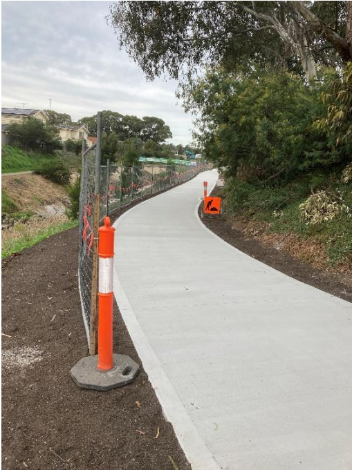
New shared path near Strathmore North Primary School (above)
