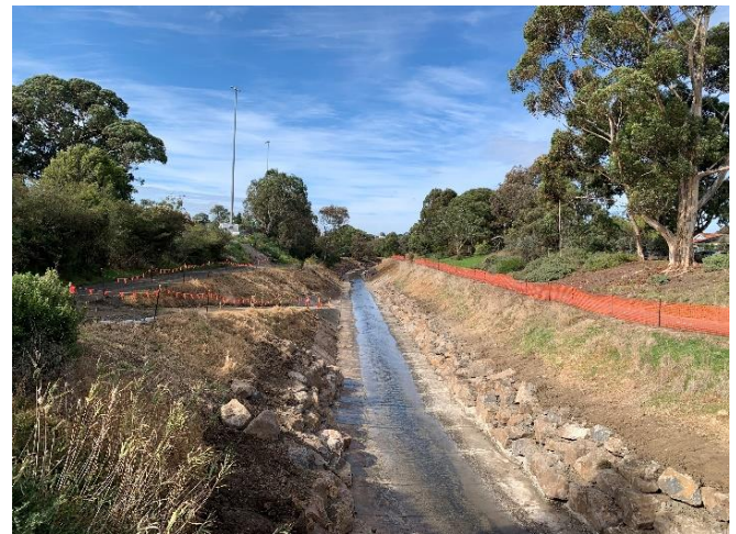
Rockwork downstream of Margaret Street bridge
