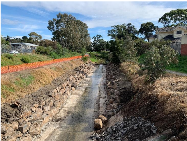
Rockwork upstream of Margaret Street bridge
