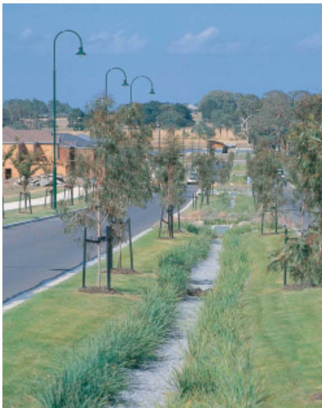
Lynbrook Estate in the City of Casey is a working demonstration of water-sensitive urban design.
