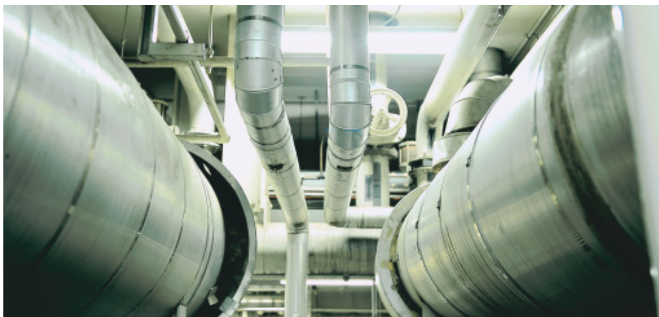
The outfall pumping station at Eastern Treatment Plant is to be upgraded as part of the Eastern Green Energy Project.
