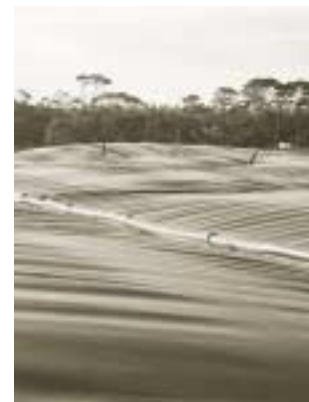
Lagoon covers at Western Treatment Plant reduce greenhouse gas emissions by trapping methane which is used to power the plant.
