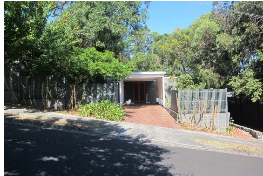
Figure 35. Modern house in Studley Park, Kew. (Context)
