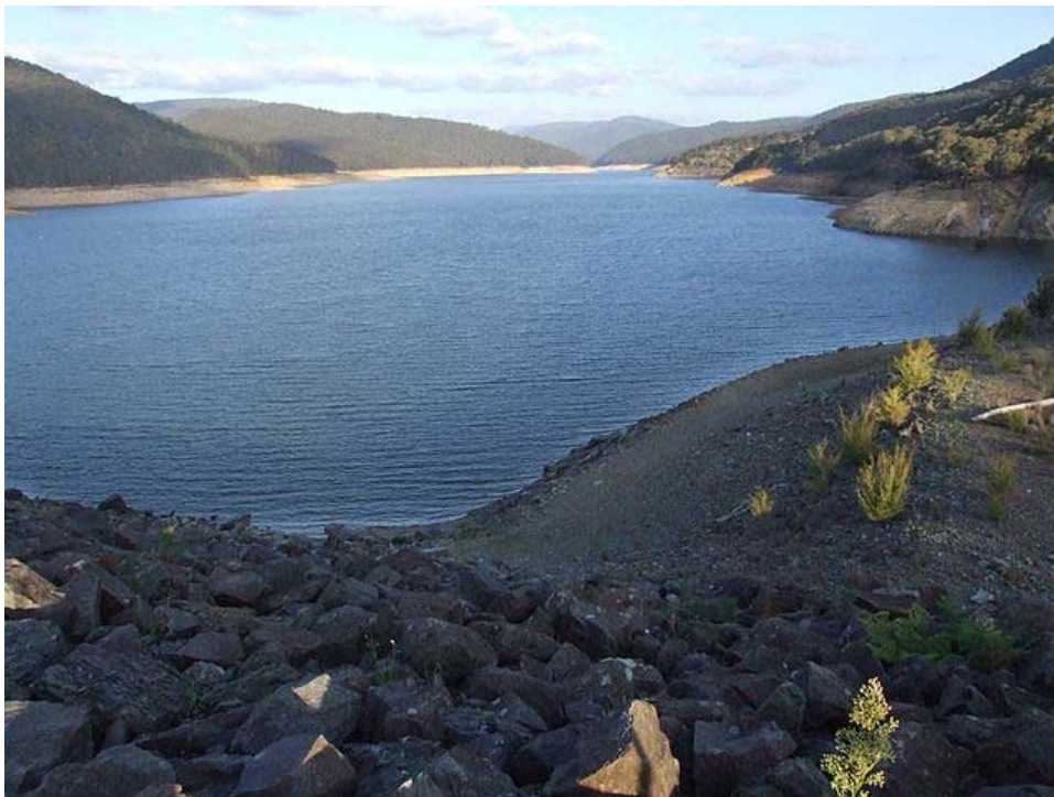
Figure 55. Upper Yarra Dam, 2007. (M1rtyn at en.wikipedia)
