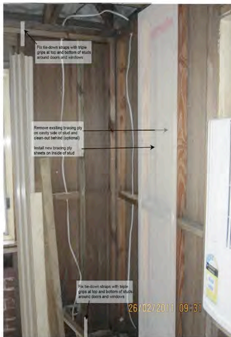
Recommendation: Bracing & Tie-down
