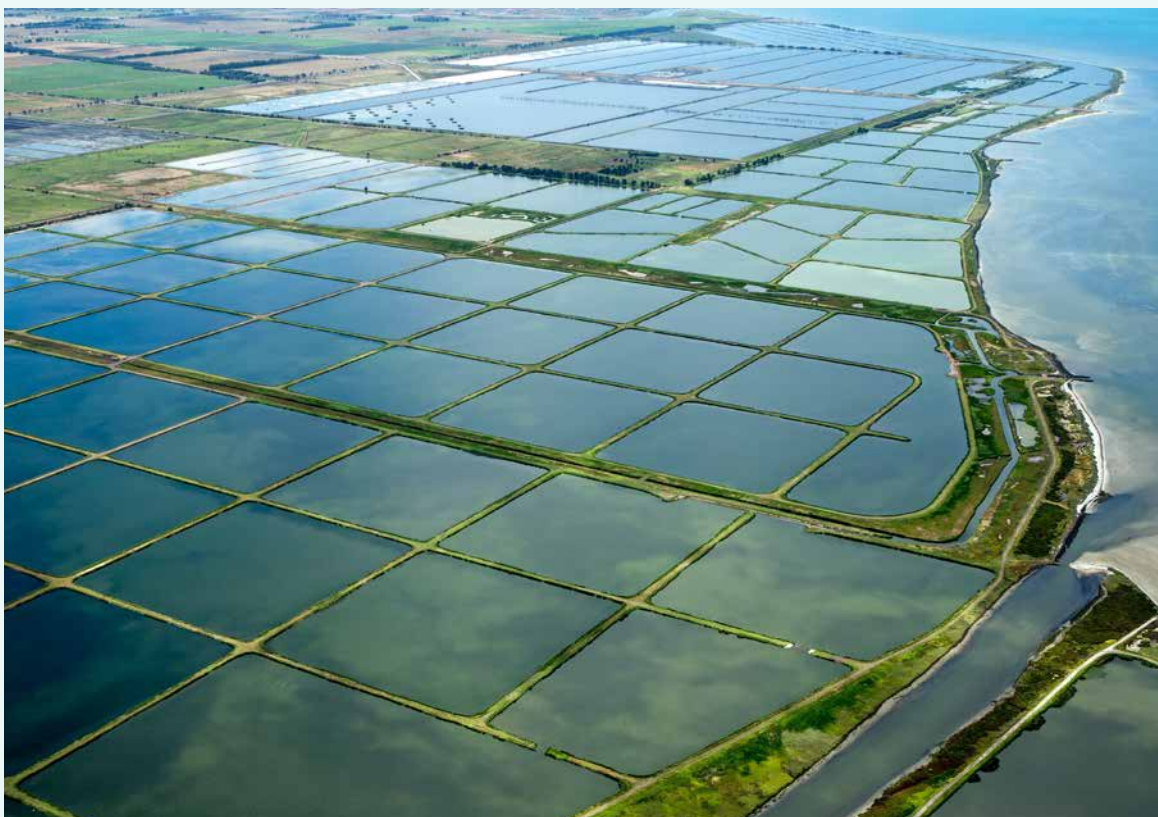
Aerial shot of Western Treatment Plant lagoons
