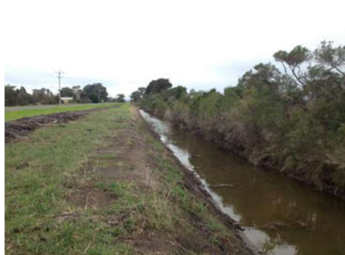
Figure 5: Dalmore Road Precept Drain
