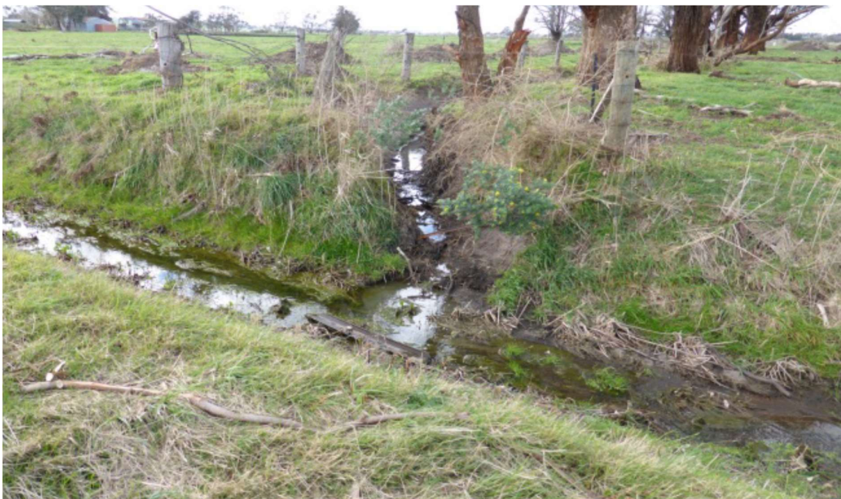
Figure 6: Private drain intersecting a Precept Drain
