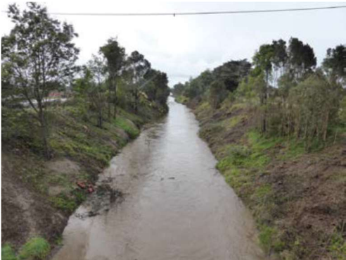
Figure 4: Bunyip Main Carrier Drain
