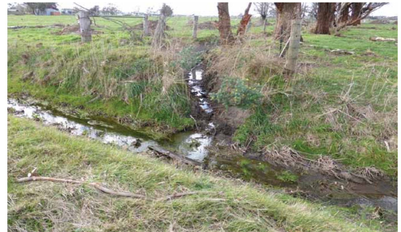
Private drain connecting into a precept drain
