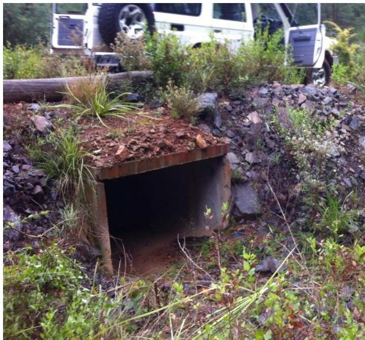
Figure 4. Box culvert under the Pipeline Vehicle Maintenance Track, Toolangi State Forest.
