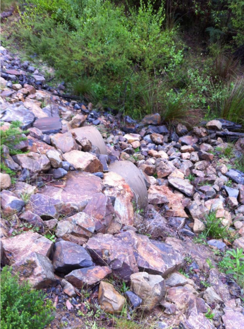
Figure 12. Rock jumble at the entrance to an underpass (dual pipes) beneath the Pipeline Vehicle Maintenance Track, Toolangi State Forest.
